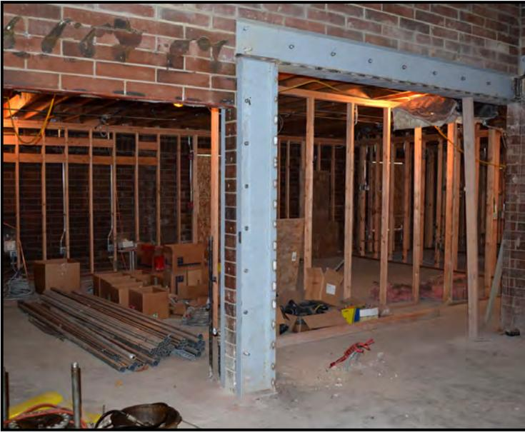
**The remodel project repairs previous seismic damage and retrofits the building to current seismic standards.**
